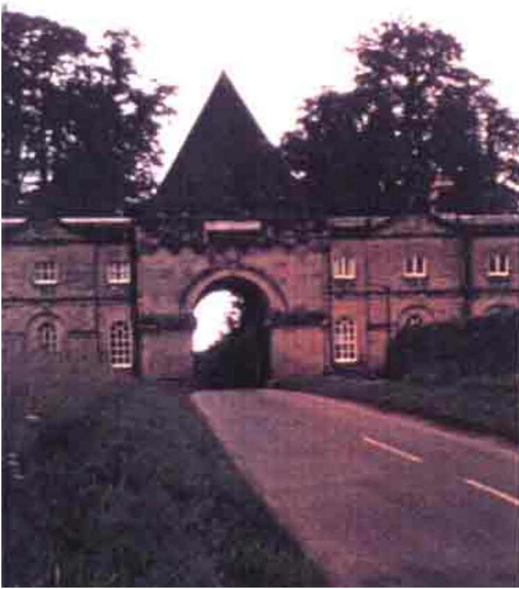
18 Castle Howard Entrance gateway by Vanbrugh
